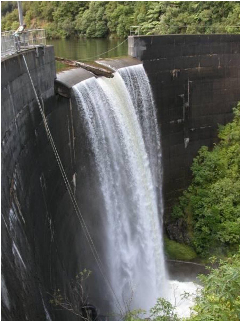
Figure 2. The 30-m high concrete gravity arch dam that forms the upper Turitea Reservoir, Palmerston North. Photo: Nicholas Ling.
